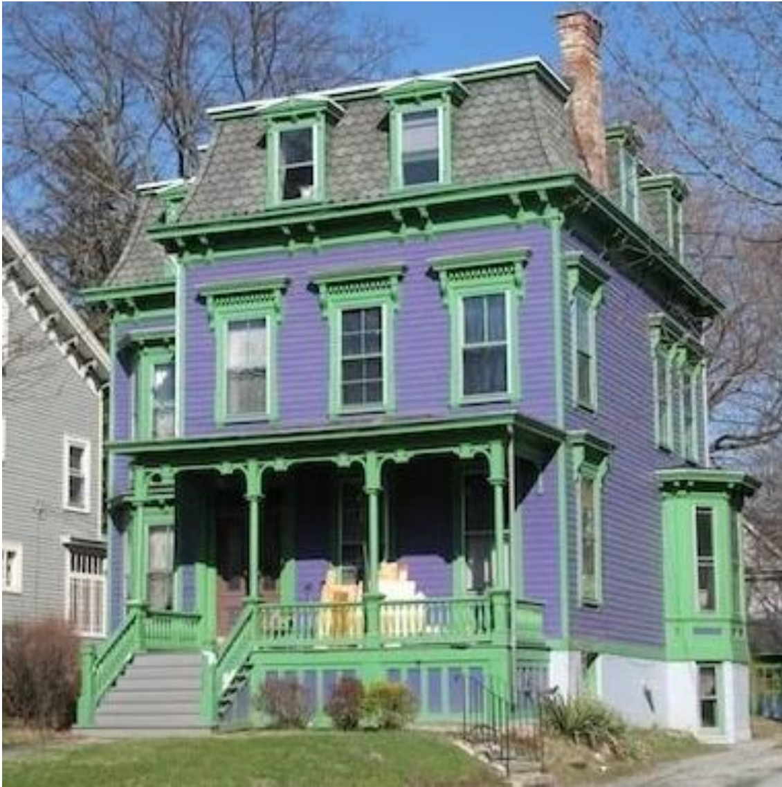
Example of structure with an arguably less than desirable historic exterior color scheme.
