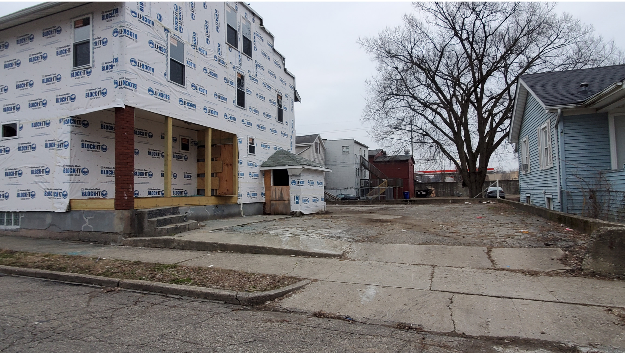
1301 Grand Boulevard Rear Facade and Paved Area
