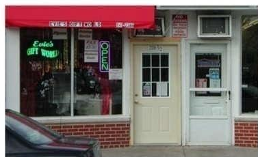
Prohibited: Residential Grade Doors on Commercial Buildings.
