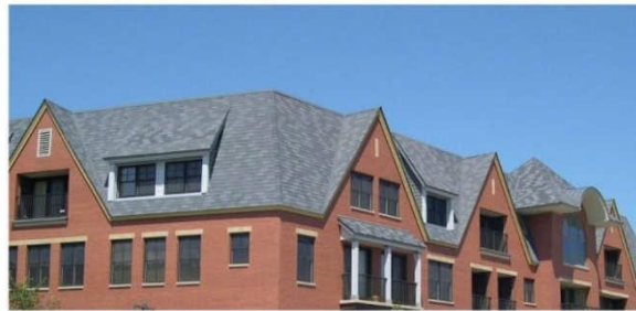
Roof Materials: Asphalt Composite Shingles
