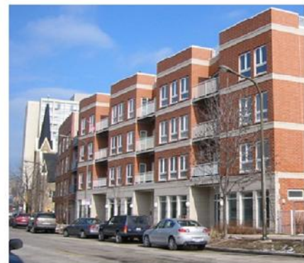
Figure 1129.46 (5). Balconies Integral to Facade.
