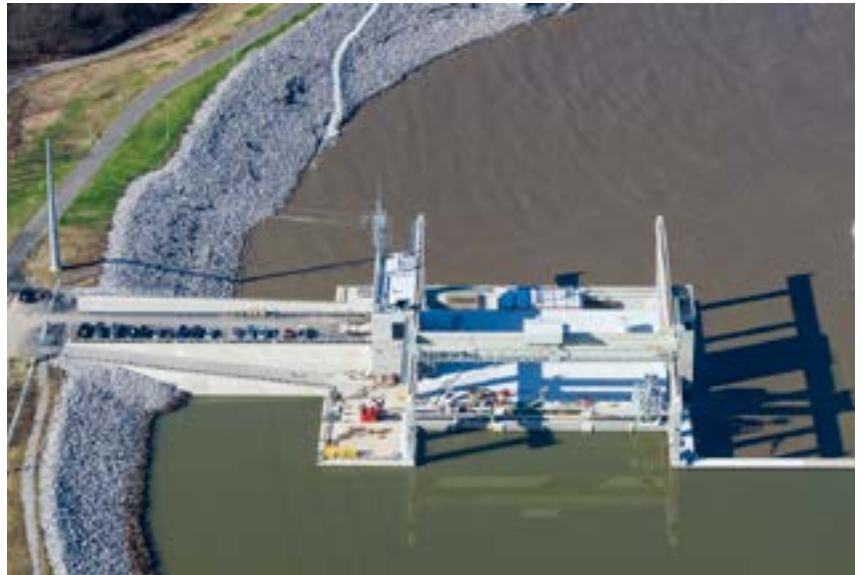
The Meldahl Hydroelectric Facility became fully operational during the spring of 2016. It is expected to generate clean and renewable energy for more than 100 years.
