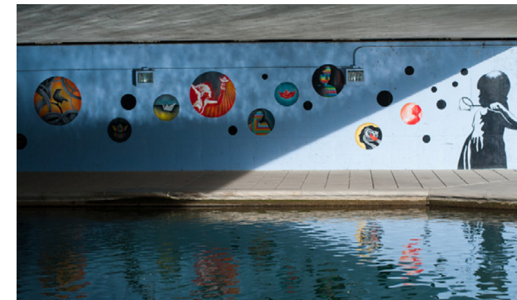
MURAL ON VERTICAL RETAINING WALL
