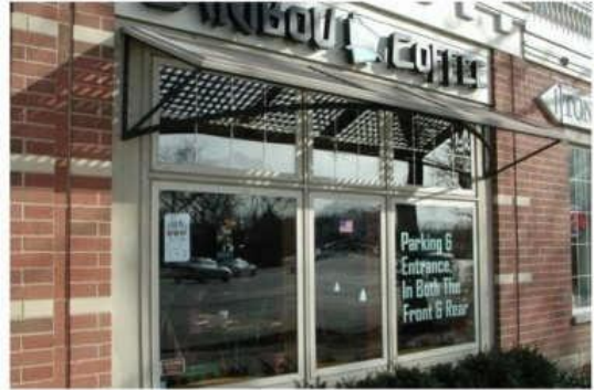
Permitted Awnings: Metal
