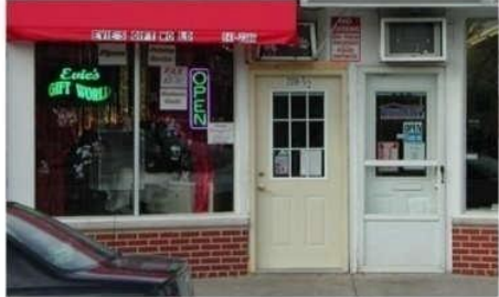
Prohibited: Residential Grade Doors on Commercial Buildings.
