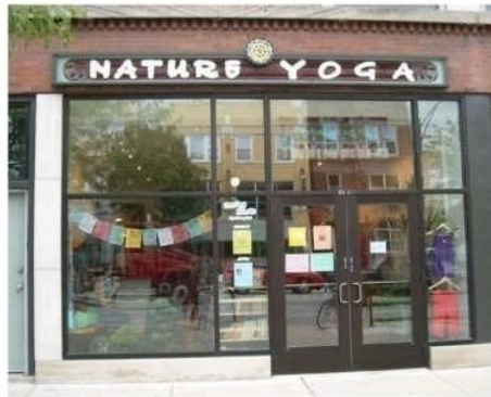
Permitted: Commercial Grade Doors & Windows on Commercial Buildings.
