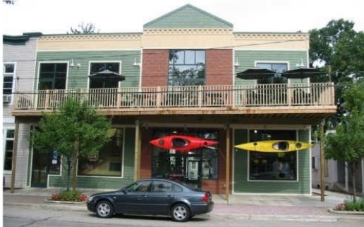
Primary Materials: Painted Wood
