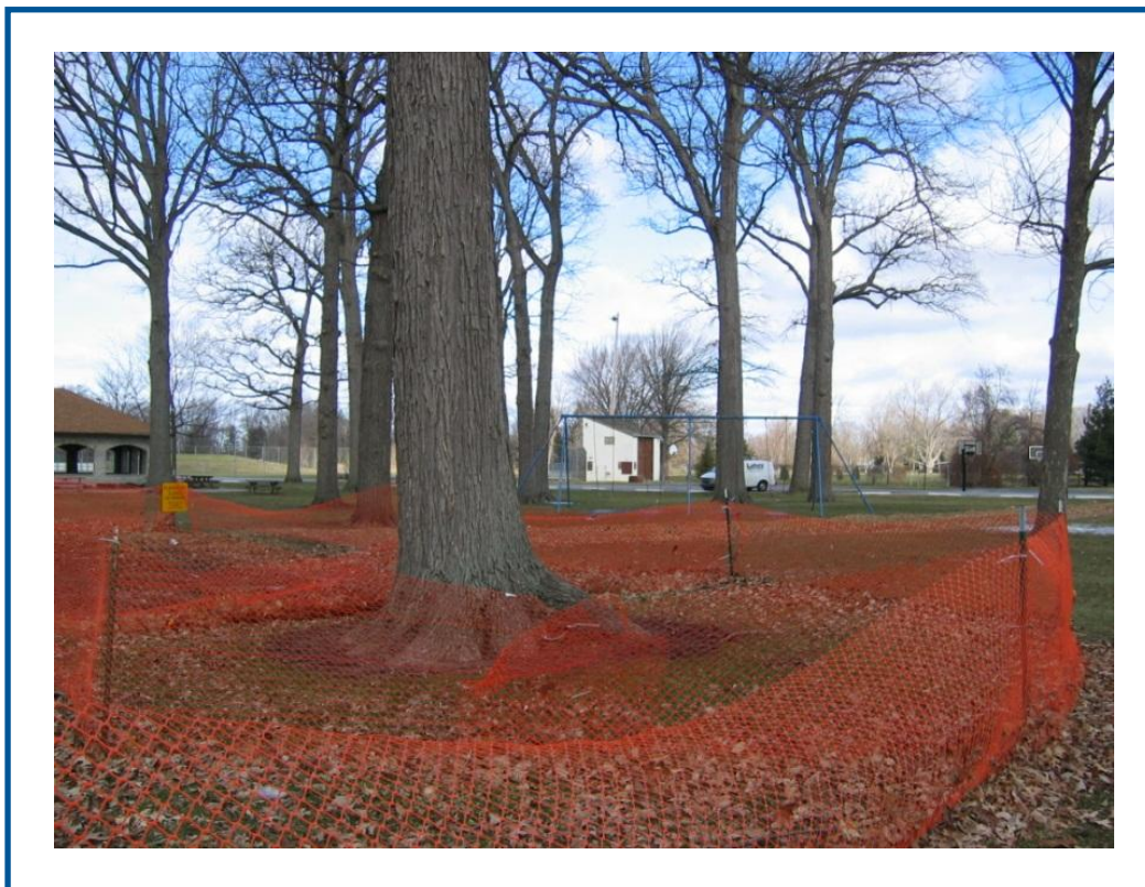
Figure 14 - Tree construction protection
