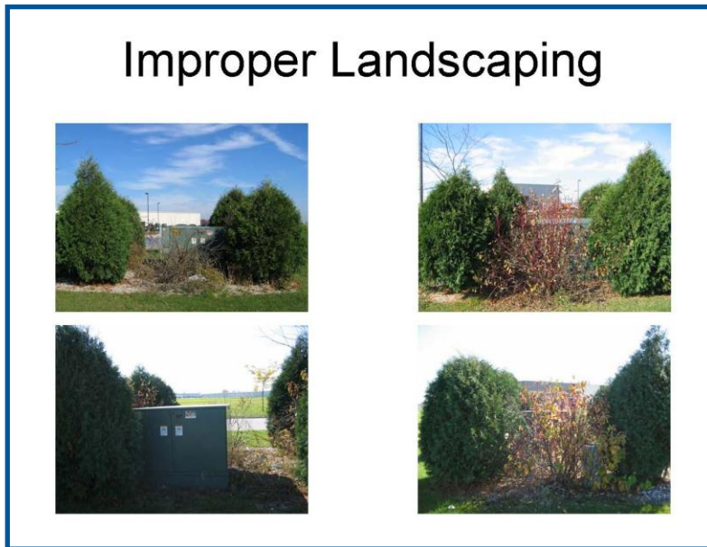
Figure 22 – Improper landscaping too close to electrical infrastructure
